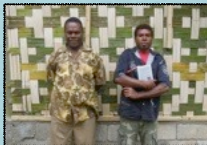
WORK: Peter and Timothy proudly pose in front of the Etas church building. They worked hard cutting, splitting, and weaving the bamboo walls the day before.
