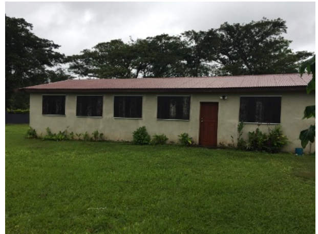
Vila building prepped and ready for Cyclone Donna. There was significant damage done in Torba Province in northern Vanuatu, but much less on us in the central and southern regions.
