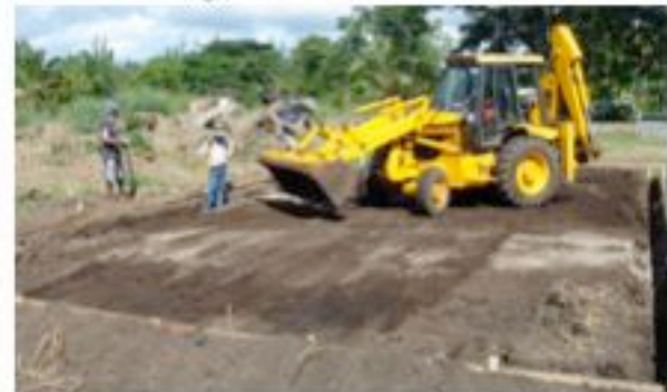
Above: The ground during construction
