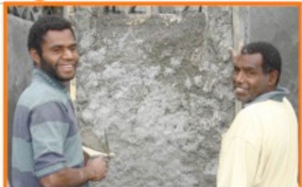
Above: Tom (L) and Patrick (R) work on plastering the toilets.
